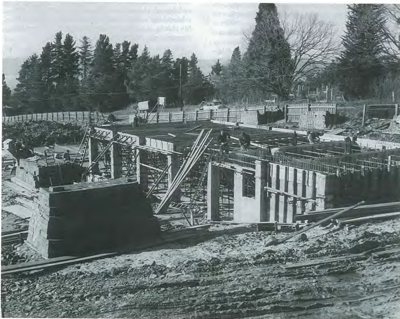
The 'new' Junior School under construction, 1956
