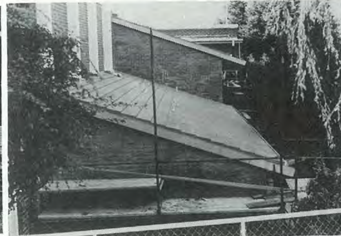
An extension to the Kindergarten, enclosing toilets and a reading area.
