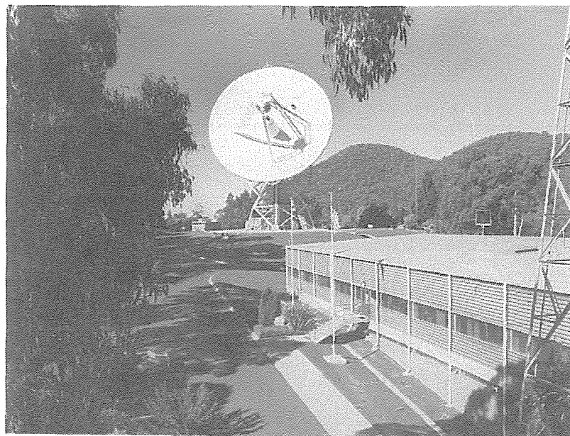
The 26 metre antenna and operations building at Honeysuckle Creek.
