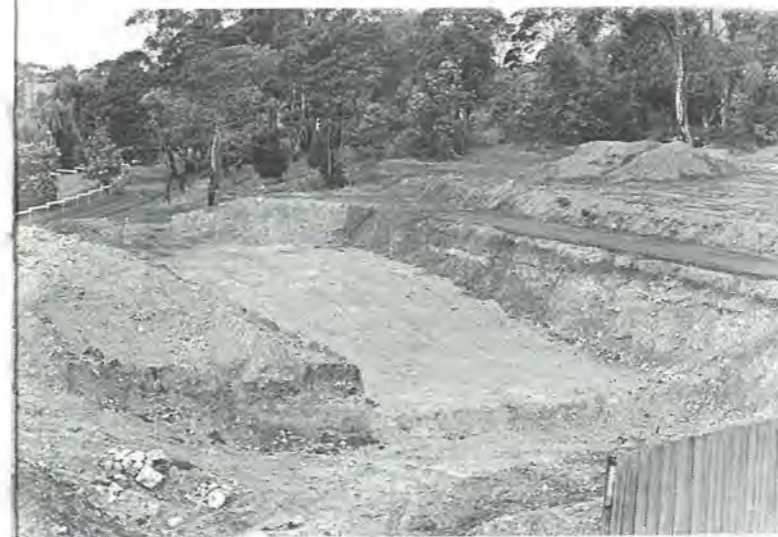
Excavation for Pool
