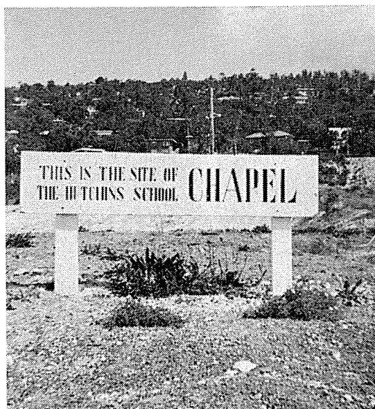
THE SOUNDS OF EXCAVATION DRAW NEARER!
